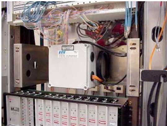
5 CARD SHELF INSTALLED IN MOUNTING BRACKET
